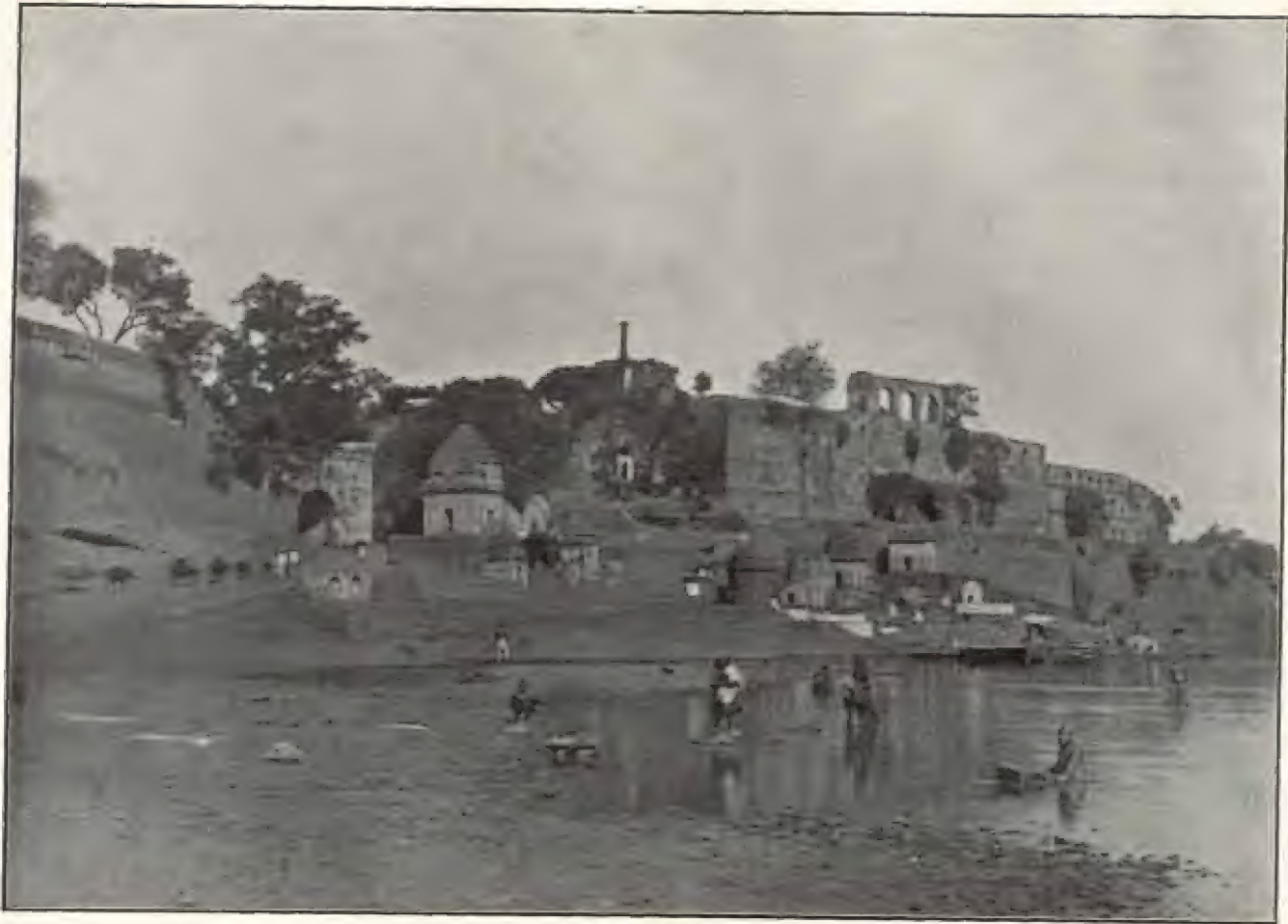
a. GENERAL VIEW OF THE FORT, RIVER SIDE, AT BURHANPUR, DISTRICT NIMAR.
